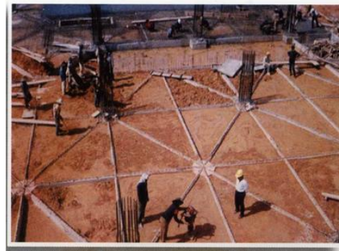
(b) The compaction of filled soil
