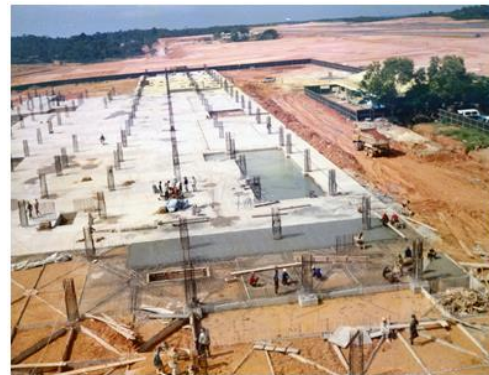
(c) The raft plate construction
