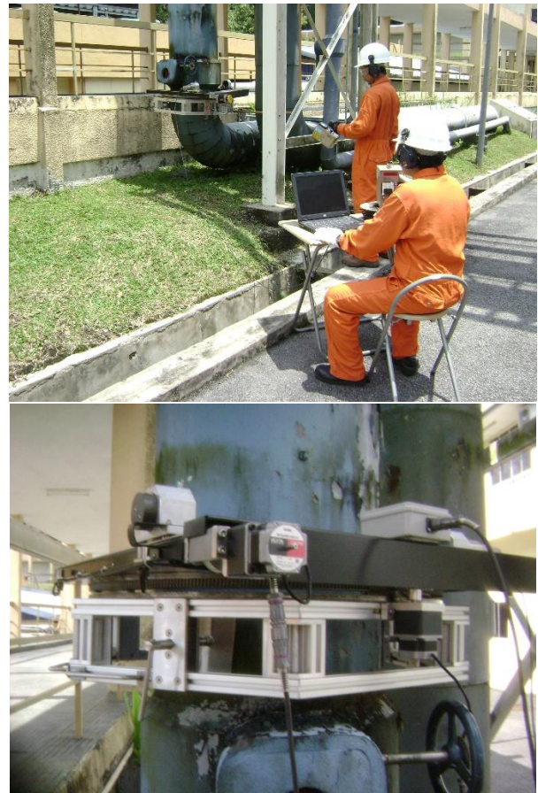
Figure 3 GammaSpider, a portable-clamp-on gamma-ray tomography system installed on a pipework
