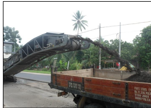
Figure 4 Cold milling process
