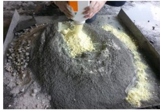
Figure 5 Adding sulfur powder into concrete mix
