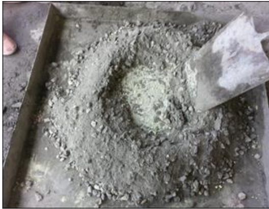
Figure 6 Manual mixing of concrete with sulfur content
