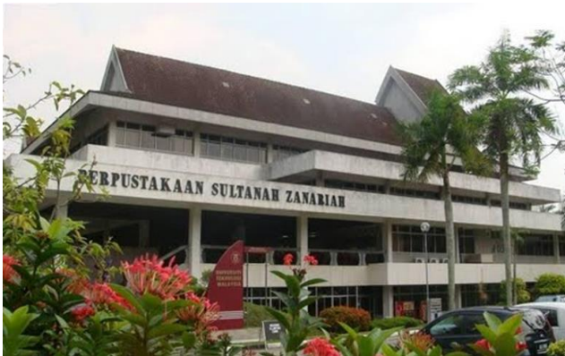
Figure 2 View of the library building
