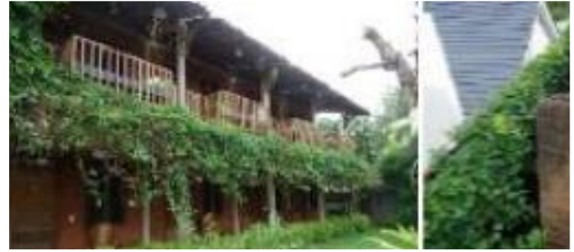
Figure 5 vertical garden in the front (left) and back (right) of Djajanti's House
