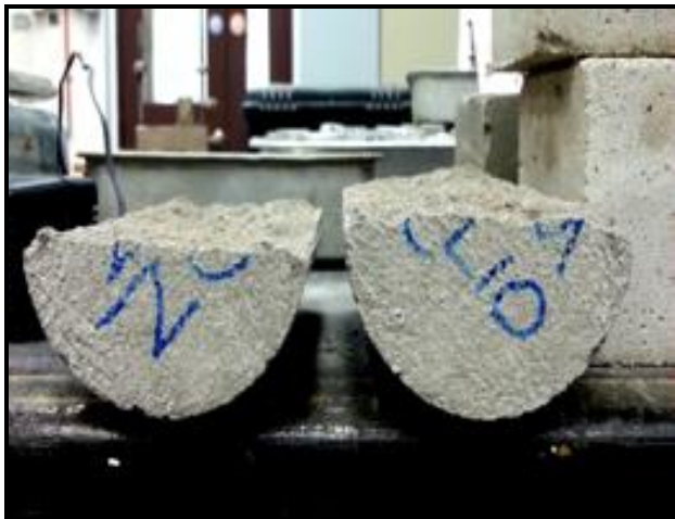
(b) Cracks formed on sample PFA-30
