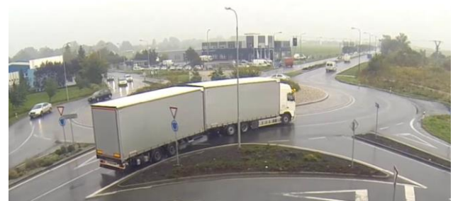
Figure 9 Incorrect passage through the roundabout with no raised lane divider.
