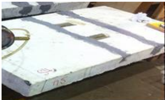
Figure 4 The crack line was patched
