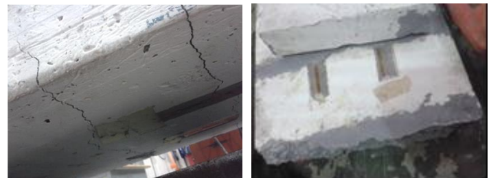
(a) Before retrofit
