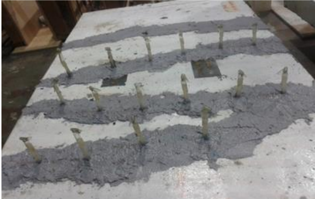
Figure 3 Installation of nozzle
