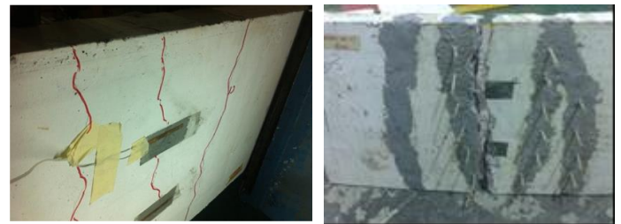
(a) Before retrofit
