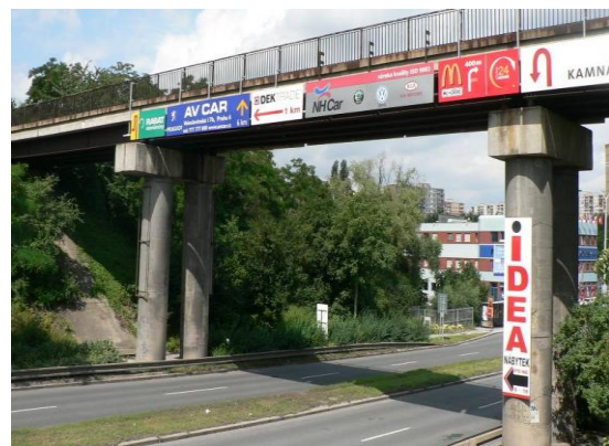
Figure 1 Side view on the railway bridge in Prague
