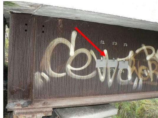
Figure 4 Southern external main girder (external web)
