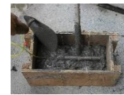
d. Placement of the concrete
