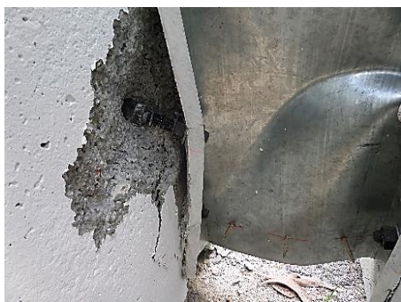
(c) Concrete crushing
