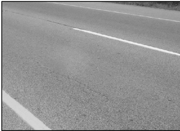
Figure 2 Second Stage of Top-down Cracking
