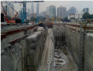
TRX Station (excavation in progress).
