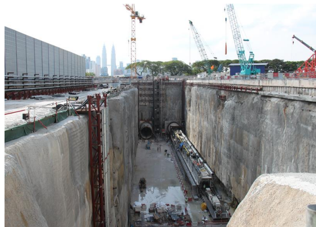
Figure 16 Cochrane Station (launching of second TBM).
