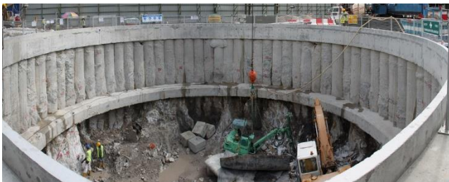
Figure 9 Circular shaft during excavation.
