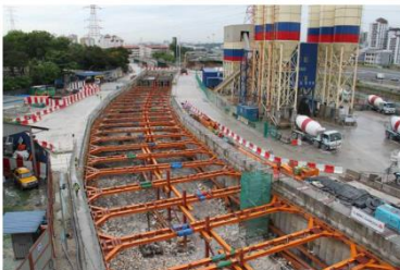
Maluri Portal (excavation in progress)
