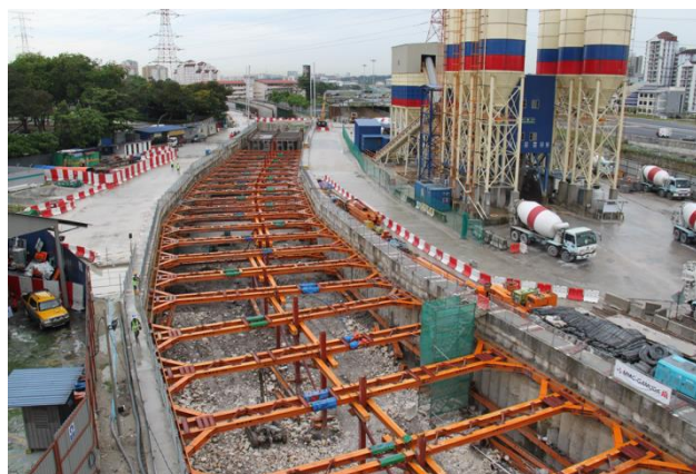
Figure 19 Maluri Portal (excavation in progress).
