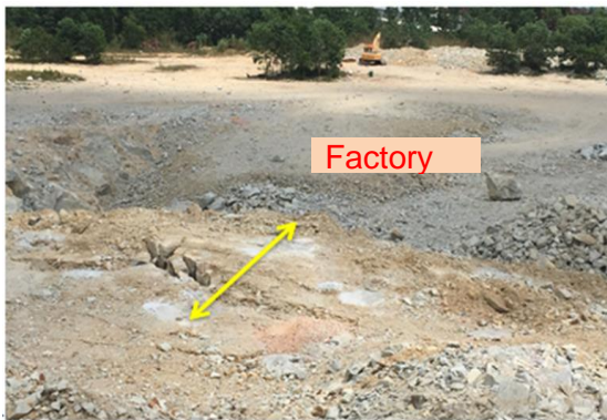
Figure 9 Status of rows of holes 2 and 3 after blast (not moved far)
