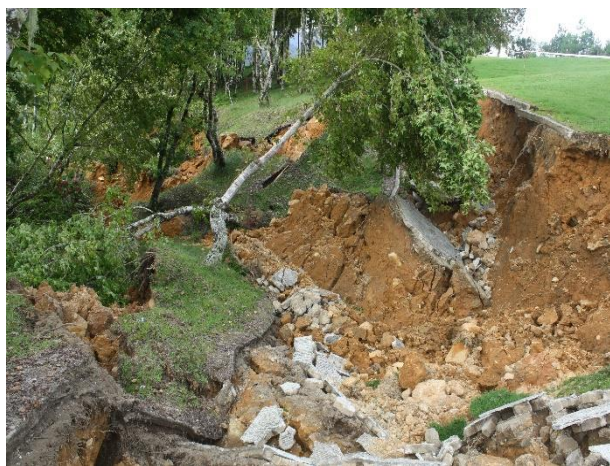
Figure 1 Ground failure after earthquake at Ranau, Sabah
