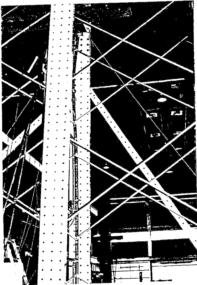
Figure 12 The buckled vertical frame at ultimate failure
