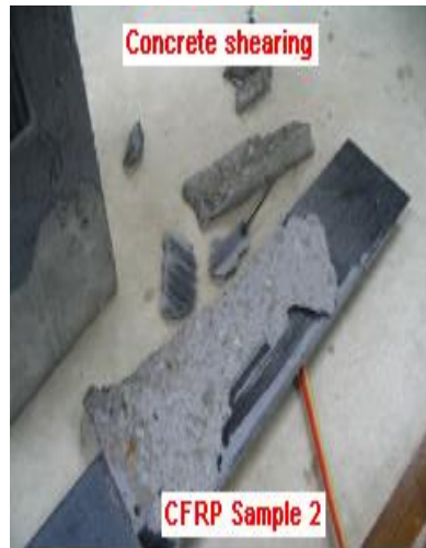
Figure 17: Concrete shearing for CFRP/Con 2
