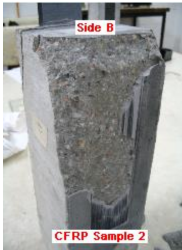
Figure 16: Typical brittle bond failure for CFRP/Con 2
