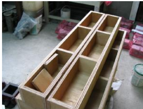
Figure 1: Formwork for concrete prisms
