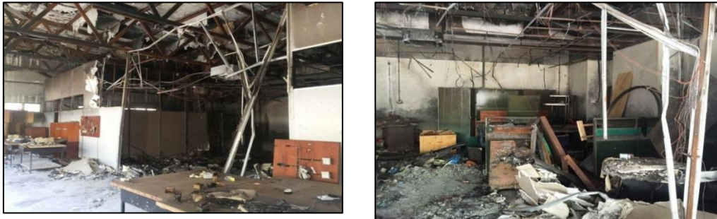
(a) (b) Figure 2: Internal views of the laboratory subjected to fire (a) From the side view of the laboratory (b) From the front view of the laboratory
