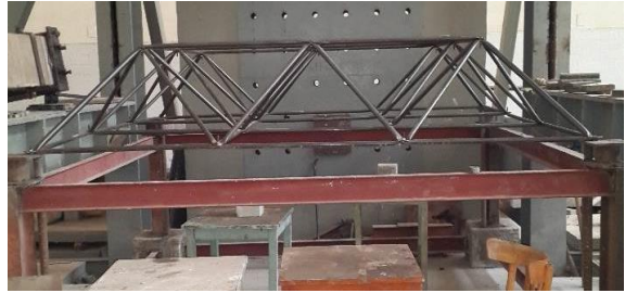
Figure 7: Assembling process of the truss#2 members
