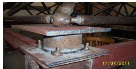
Figure 5: Connection between truss#1 and supporting frame
