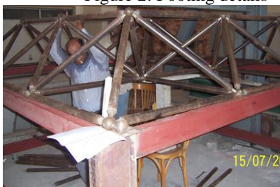
Figure 4: Assembling process of truss#1 members
