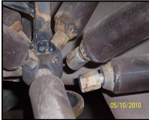
Figure 24: Collapse in connections (7&11) from the second test of truss#1
