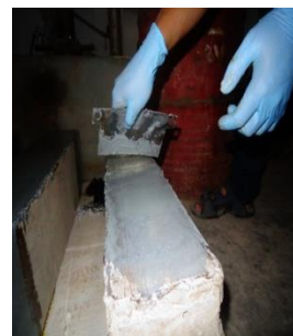
Figure 2(c) Application of putty filler on beam surface
