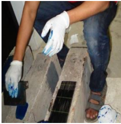
Figure 2 (g) Applying epoxy adhesives
