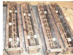
Figure 4(a) Reinforcement placed in the mould
