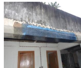
Figure 2(f) Demonstration of strengthening on an existing beam
