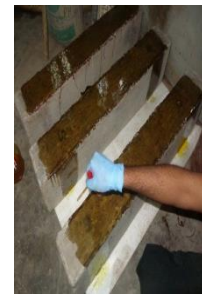
Figure 2(b) Application of epoxy based resin
