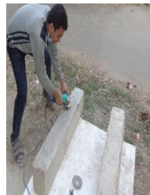
Figure 2(a) Surface preparation of beam specimen
