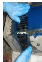
Figure 2(e) Installation of end anchorage
