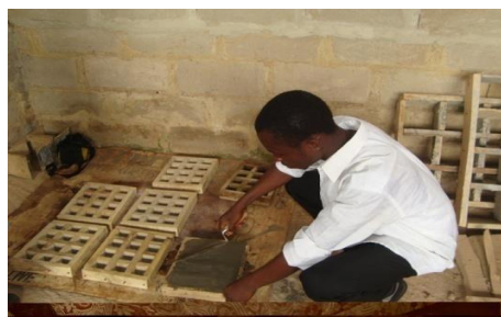
Figure 6: Filing the Mould with Mortar
