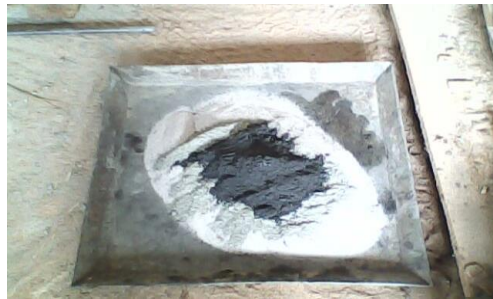
Figure 4: Batching of Mortar
