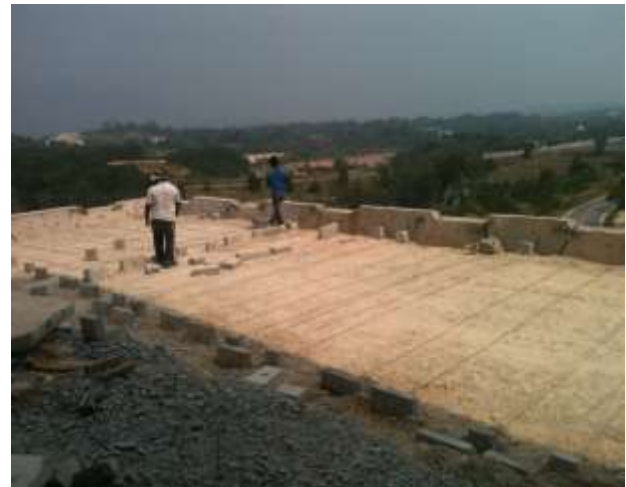
Figure 3 Dismantling and reconstruct the top panel 2m from the finished floor level to reduce the difference of verticality wall panels.
