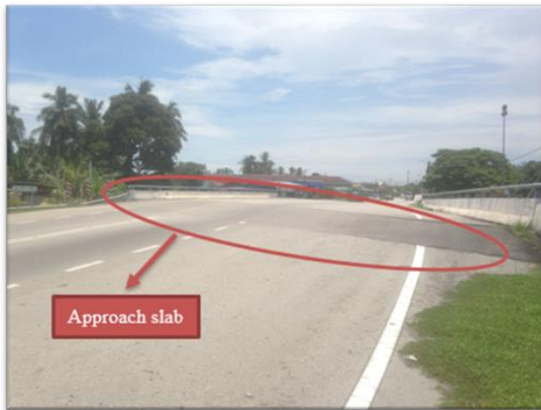
Figure 2 Approach slab at Jambatan Parit Jamil
