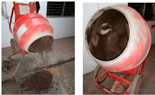
Figure 5: Machine Mixing of Concrete (Mixing concrete with a mixer machine in Laboratory)
