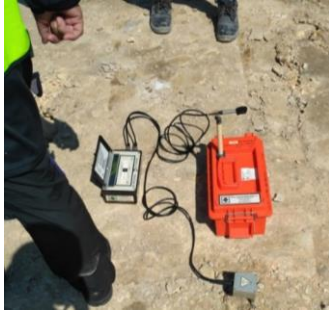
Figure 4 Instrument setup for vibration monitoring test
