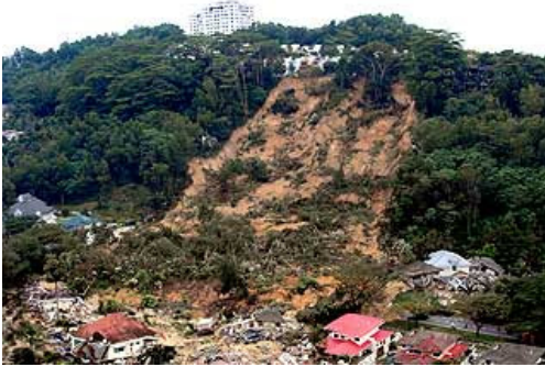
Figure 7 Bukit Antarabangsa landslide in 2008
