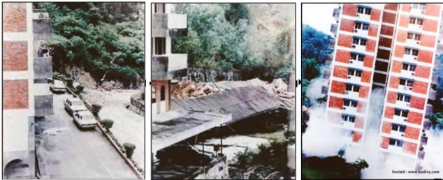
Figure 3 Highland Tower condominium collapsed
