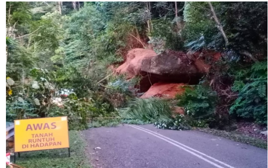
Figure 14 Rockslides at Jalan Raub-Bukit Fraser
