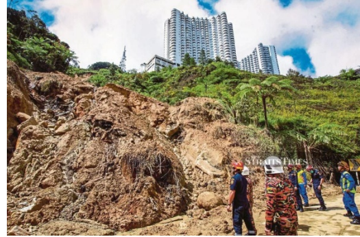
Figure 10 Landslide at Genting Highland Road
