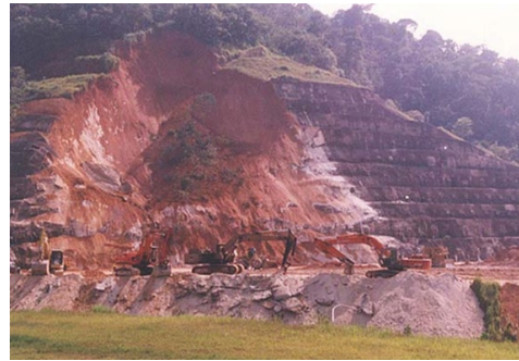
Figure 4 Close view of Gua Tempurung Landslide at North South Expressway
