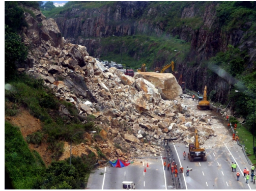
Figure 6 Bukit Lanjan rock slope failure
