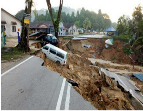
Figure 9 The scene of the 26 November 2016 Taman Idaman landslide.
