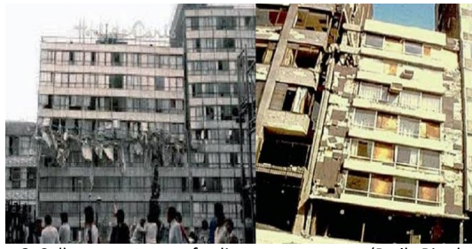
Figure 3 Collapse patterns of adjacent structures. (Patil, Biradar, and Doddamani 2022)
