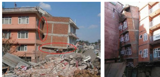
Figure 2 Collapse patterns of adjacent structures. (Rai et al. 2016)
